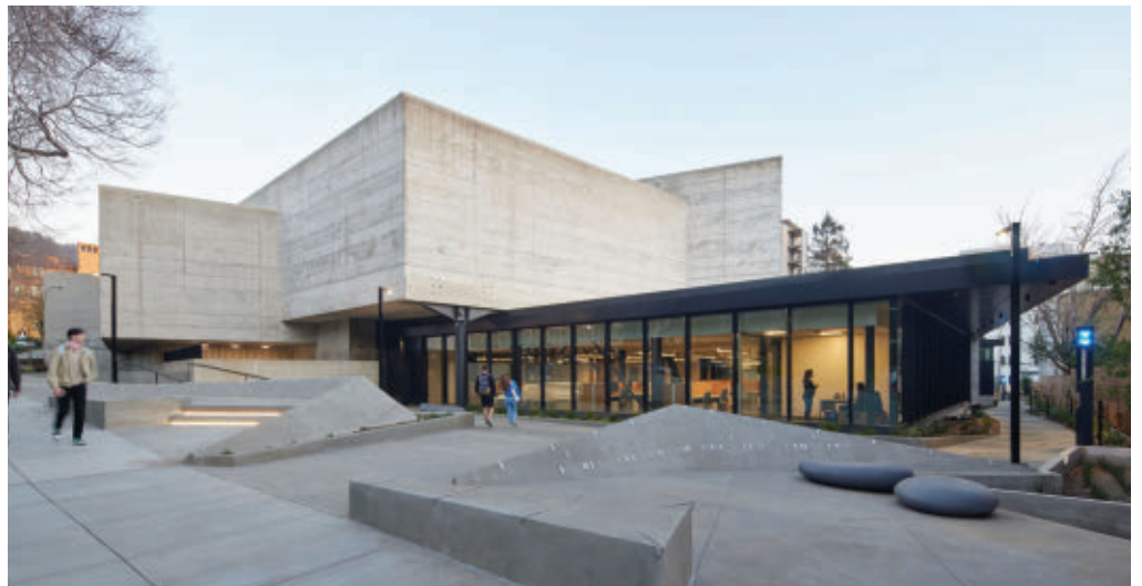
Housing the innovation Hub in this rehabbed Brutalist structure helped prevent the demolition of the 1970s-era building. MBH Architects unveiled dramatic skylights that cast light over the building’s many angles and shapes, changing throughout the day. The light fixtures assist with wayfinding and mimic the original lighting of the art museum.
